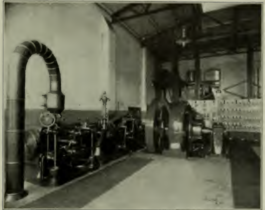
16X30 MURRAY-CORLISS ENGINE WITH 170-KILOWATT SHELL GENERATOR
